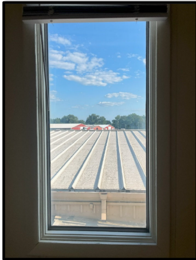
View from AGR building breakroom 113
